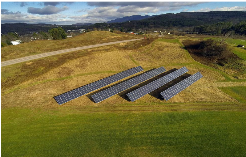
Solar array in Duxbury, Vermont developed by Green Lantern Group for Crossett Brook Middle School
