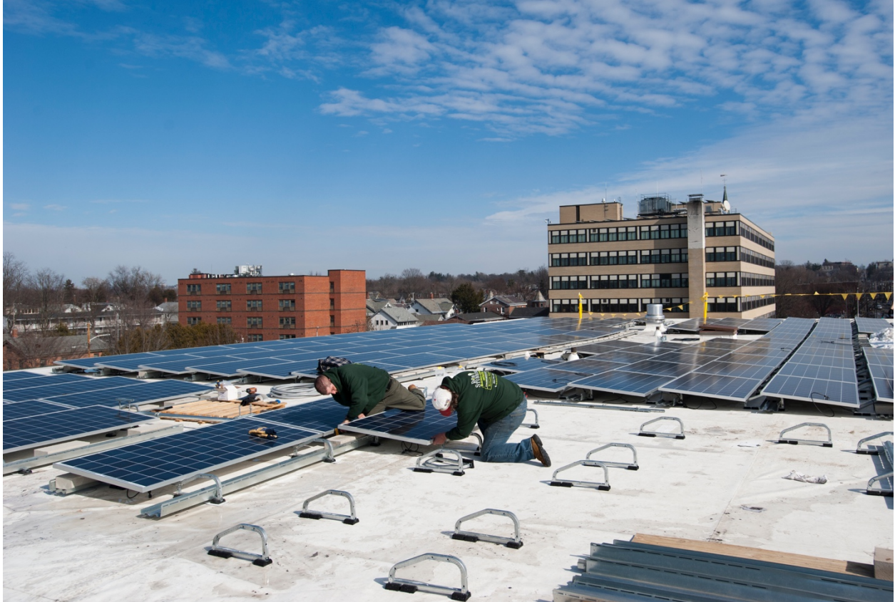
SunCommon installers mount panels on flat roof in Downtown Burlington, VT
